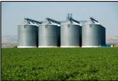
Grain Storage Facility
