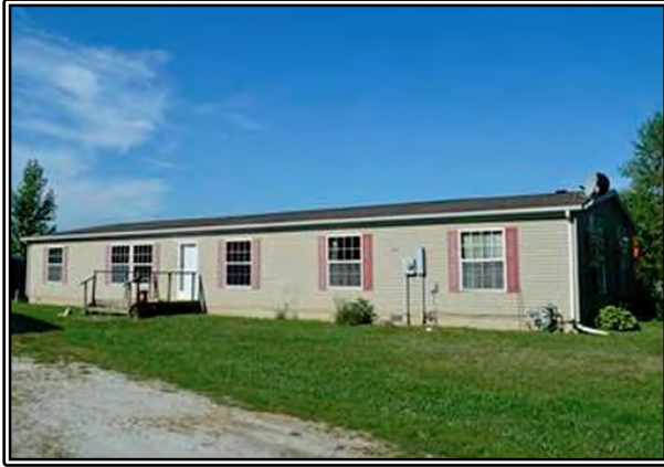
713 South Lafayette Street
